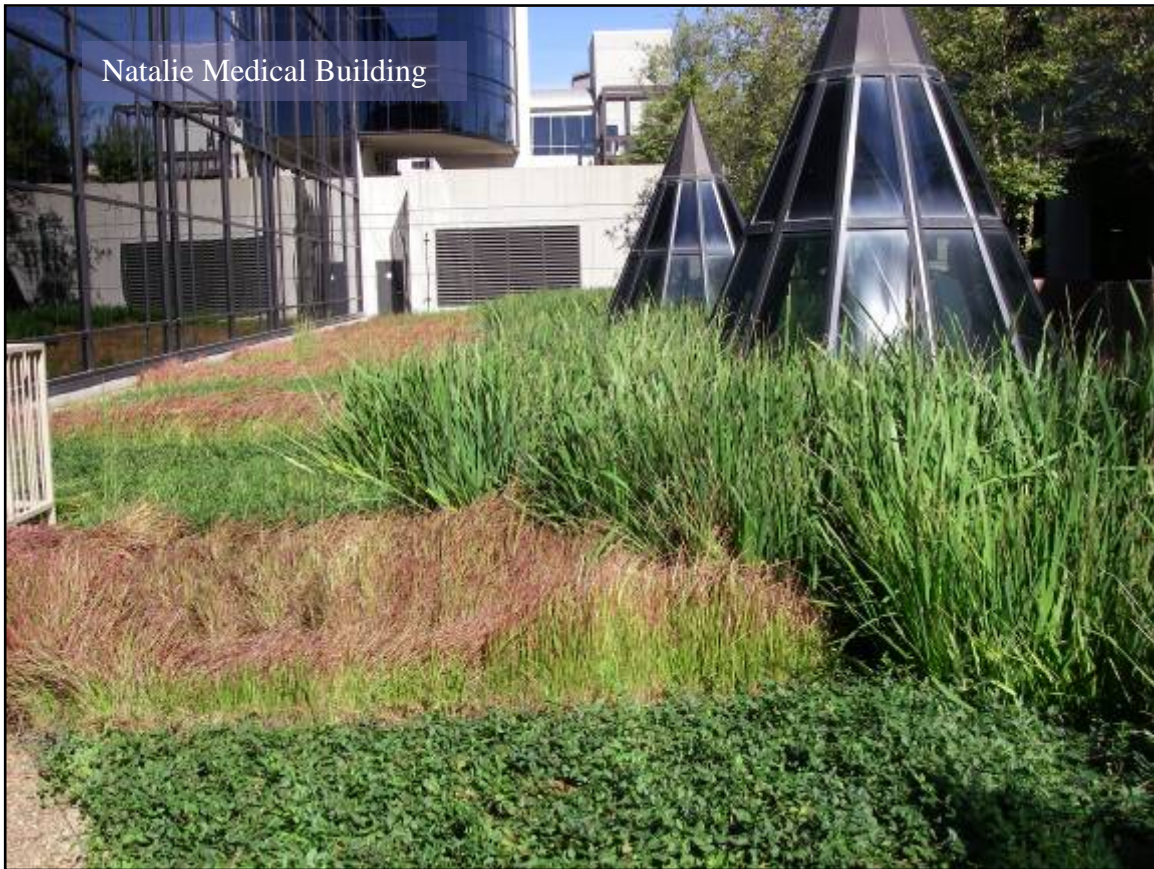
The Natalie Medical Building, (6475 S. Yale, Tulsa, OK) managed by Warren Professional Building Corporation, has a very nice green roof with conical skylights
