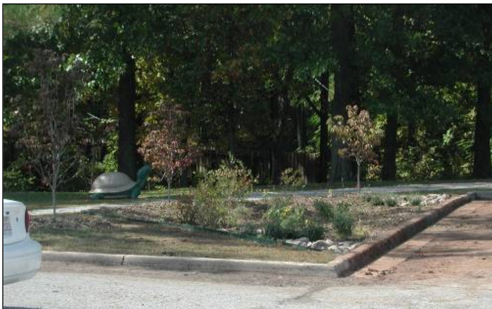
Figure 2: Rain Garden built in Broken Arrow at the Ray Harral Nature Center. Curb cuts will be Made in 2011 once the vegetation is better established. Outflow notches already exist.
